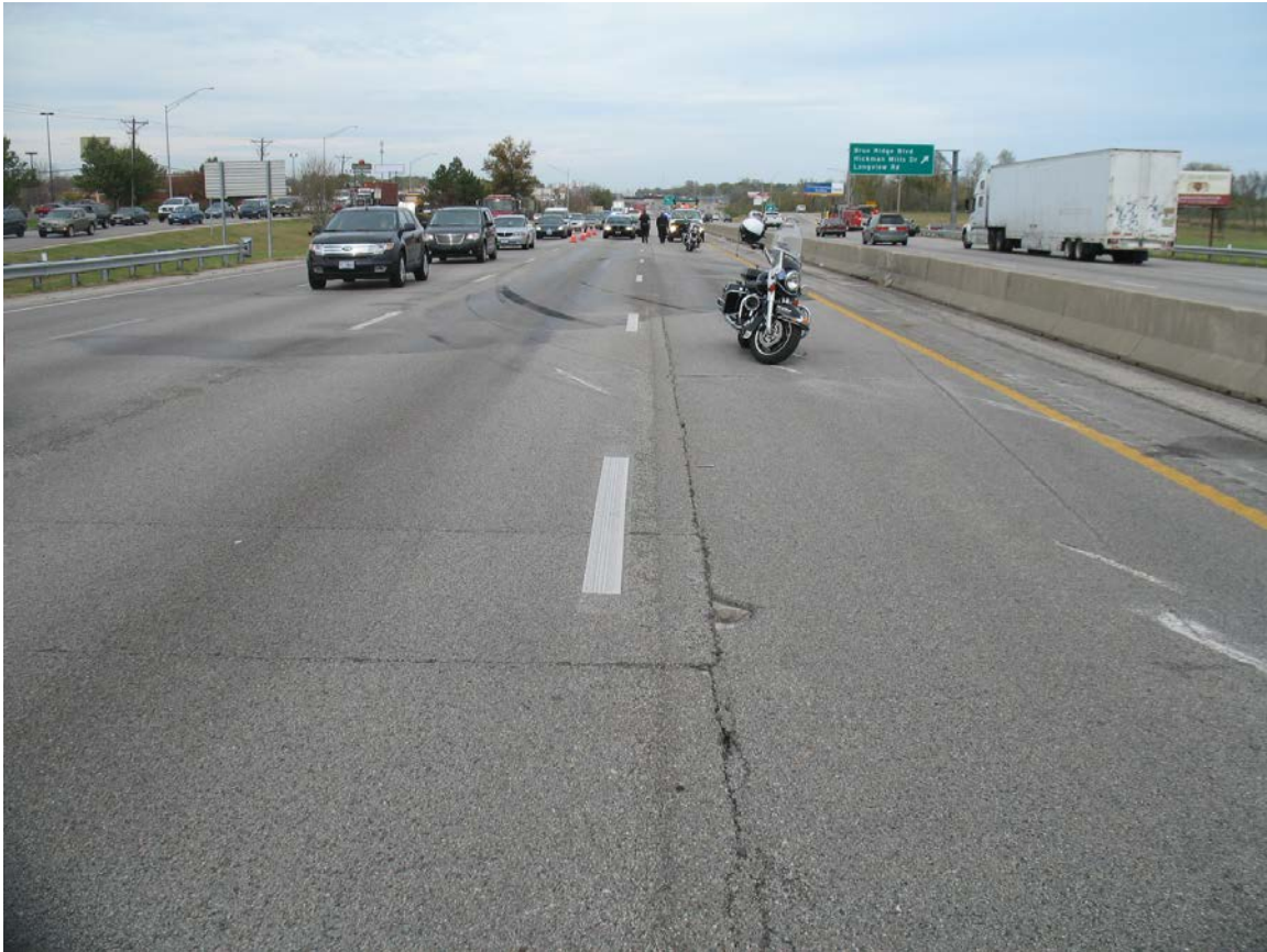
Figure 10 Police IMG 3514 Looking north
